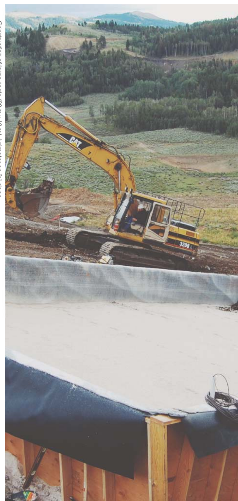
Construction of large-scale (20 m x 10 m) lysimeter on 3:1 slope.
